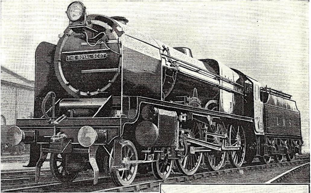
The Royal Scot, England's most famous train, is on exhibit at the Century of Progress. British locomotives cannot approach American engines in size because of restrictions as to clearance and size made necessary by low bridges, etc.
