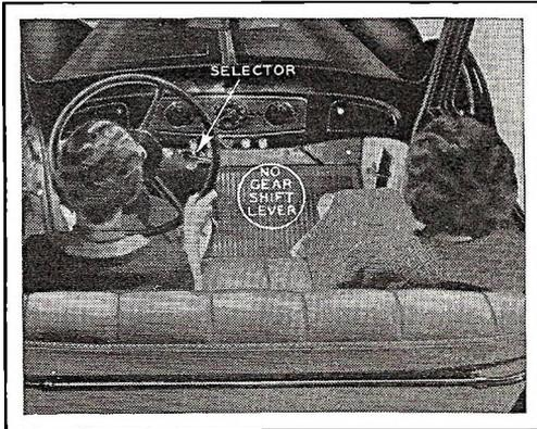
To start popular new car without gear shift lever, driver simply moves the selector on the dash, releases the clutch and steps on the gas. "Low," "second" and "high" is then thrown in automatically as the car gains speed.
