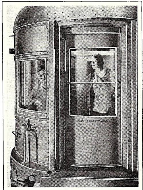
Rounded end of new Pullman car, interior of which is shown on opposite page. Steel, too heavy, is out of the picture in new railcars; light metal alloys take its place.
