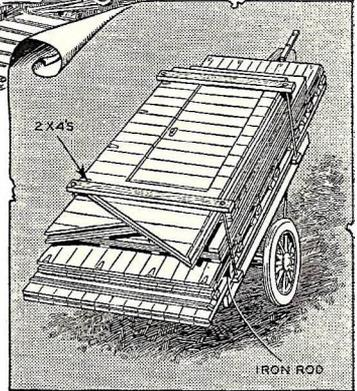
Units of house are transported on trailer to camp site. 2x4's underneath and on top are joined by iron rods to clamp the units into an easily shipped bundle.
