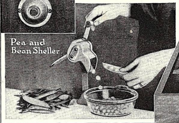
Labor of shelling peas is reduced to absolute minimum with this automatic sheller now on market. The peas are fed into the hopper with the left hand while the crank is turned with the right. The peas or beans roll out into the dish while the empty pods drop on the other side. Clamps to table as shown, and does a clean job of removing strings and separating peas and pods.
