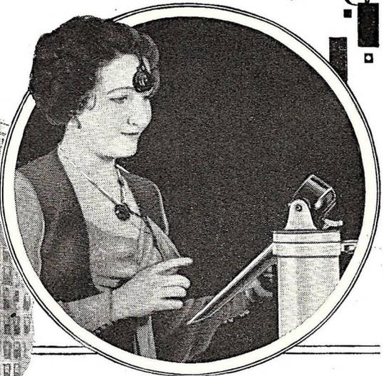
Broadcast technique of singers is greatly improved by small auxiliary microphones, placed over nose sinus and chest. It is unnecessary to "hug" the mike during performance.
