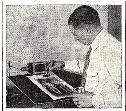
Brush on developer using swift vertical, horizontal strokes.
