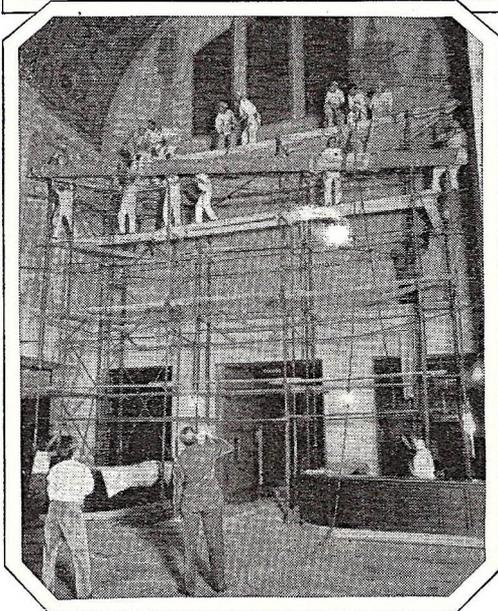
In hanging the murals, they were hoisted in rolls by black and tackle, anchored at the top, and bound to the wall with white lead against which the canvas was flattened while the lead was still wet. Note intricate scaffolding employed.
