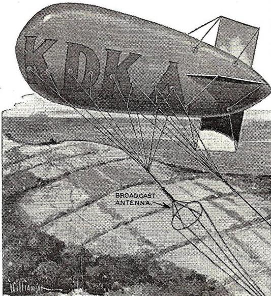
Artist's drawing illustrates how vertical antenna was suspended from captive balloon to test directional qualities. Electric winch shown in top photo, paid out and reeled in cable.
