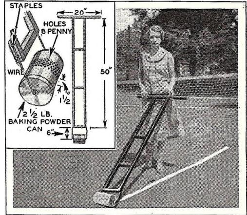
Marker is assembled as illustrated in the drawing. Can is filled half full of air-slaked lime, free from lumps, and rolled over the court like a lawn mower, leaving straight line.
